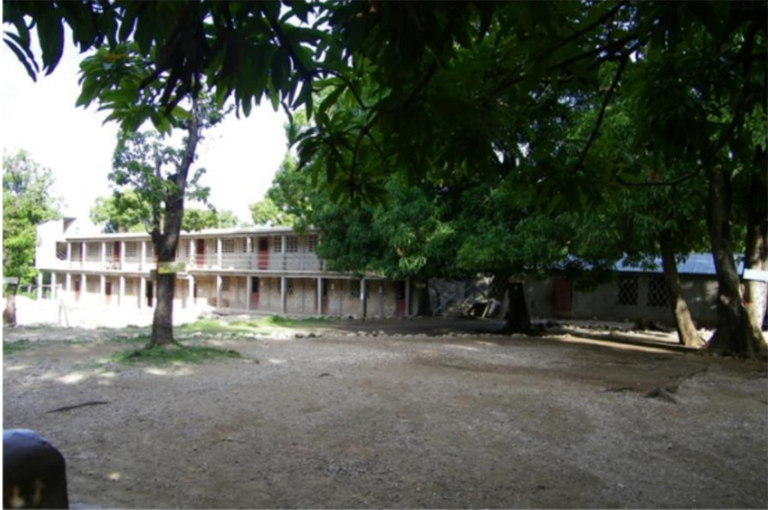
Main School Bldg - Kitchen at Right
